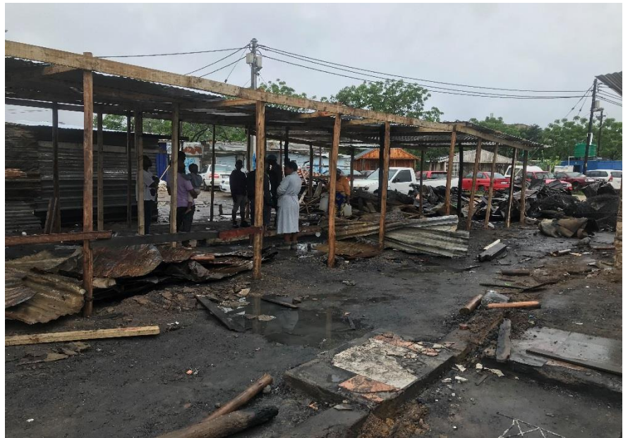
Communities rebuild after a devastating fire in Parkington in 2021
