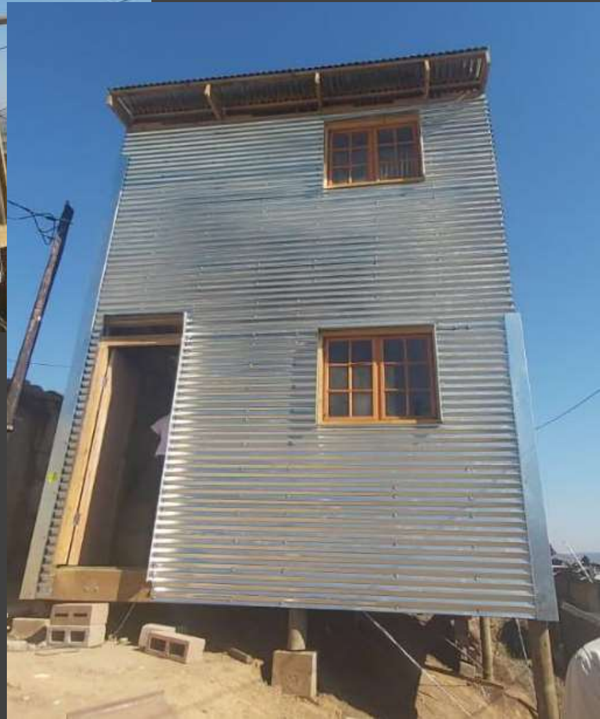
External cladding being installed
